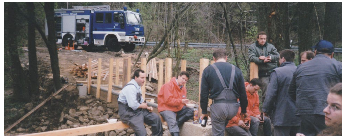
Brückenbau in Roetgen 1999
